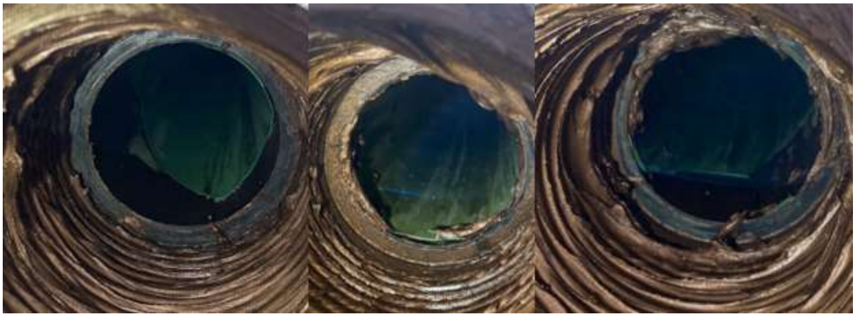
Figure 8: Drill pipe joints laid down with ID coating defects
